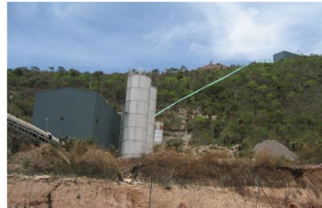
Depiction of the DSI GPS that was abandoned due to geological instability.
