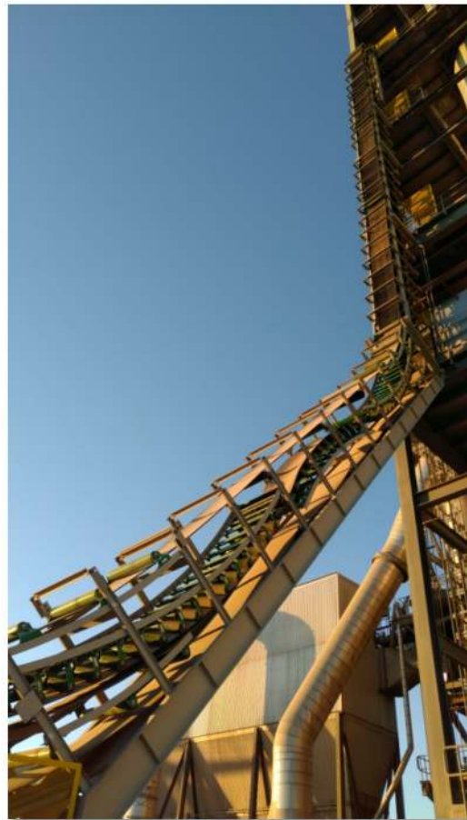
Figure 2: DSI Snake/GPS Conveyor Tire Chip 90° Elevation along building
