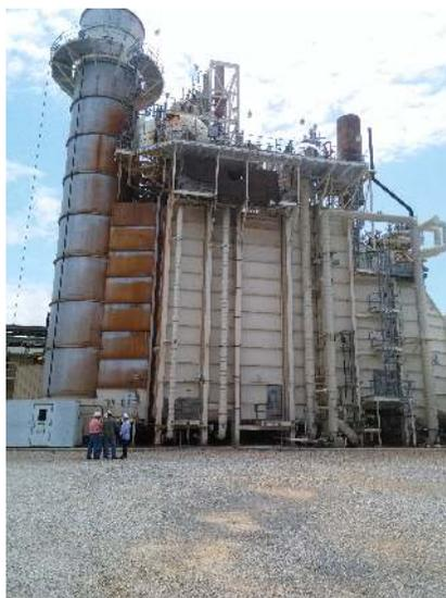
**Figure 1: HRSG (Heat Recovery Steam Generator)**
