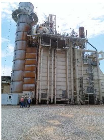
**Figure 1: HRSG (Heat Recovery Steam Generator)**
