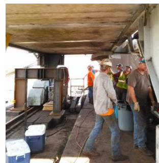
Figure 2: Temporary steel support
