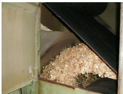
Chips discharge gently and cleanly from the conveyor.
