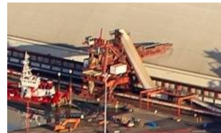
Figure 2: Sandwich Conveyor fed by low-lift tripper
