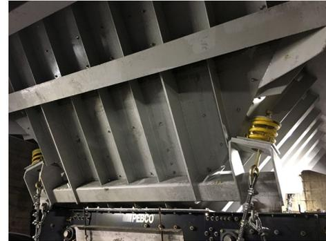
**Figure 1: Hollow structural sections used to resist moment and torsion created by new feeder loads.**
