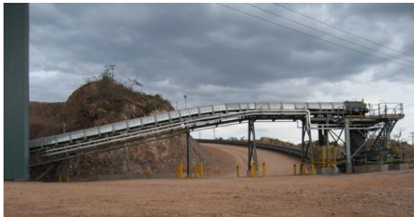
Looking up the Overland Path: From TB25 to TB26 Looking Up
